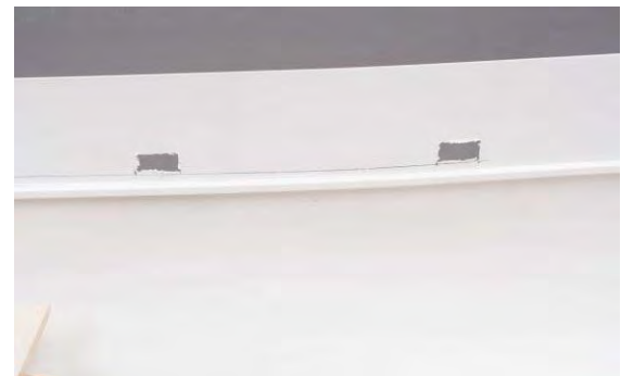
Fig. scuppers cut out, from inside
